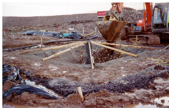
Figure 5 Completed experimental liner system prior to filling and fitting of the rain cover
